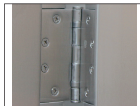
Fully Mortised Hinges Flush mortised hinges provide a clean and smooth finish to the door.
