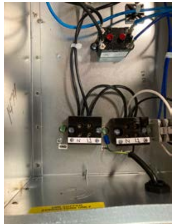
Figure 10: Jumpered Electrical Terminals
