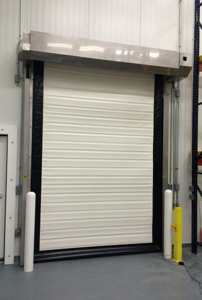
High-Speed Interior/ Exterior/Freezer Fabric Roll-Up Doors MODEL 615/615F
